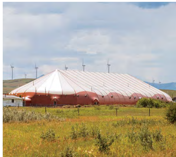
The new Multipurpose Centre on the Piikani lands in Brocket, Alberta.
