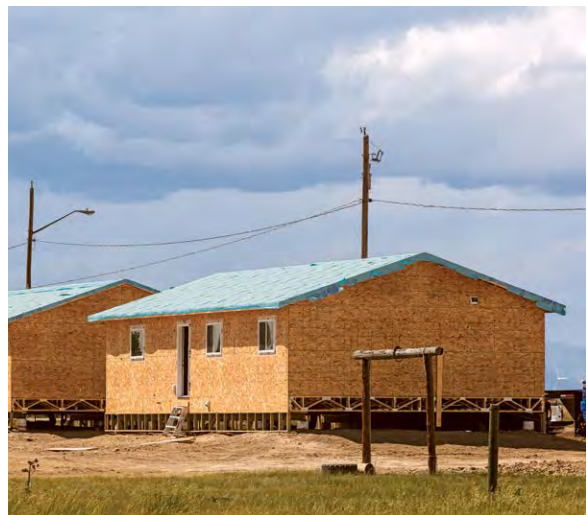
New housing being constructed on the Piikani lands in Brocket, Alberta.
